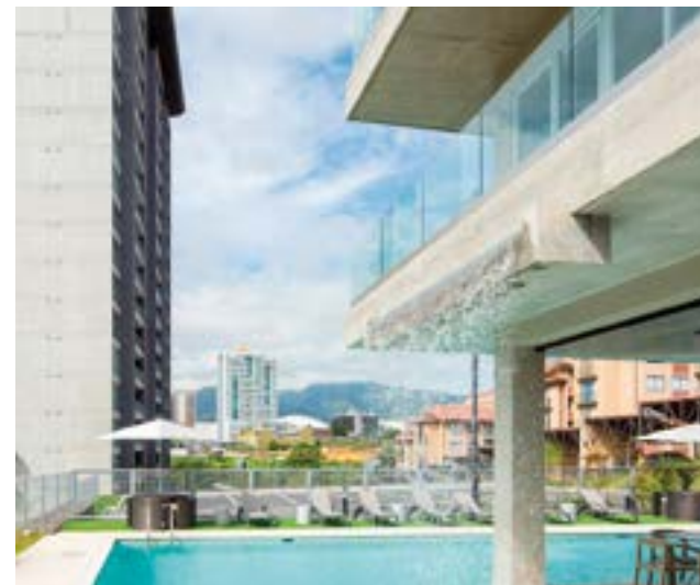
Residencial Azenza Towers. San José-Costa Rica. GlassFit SV-1301.
