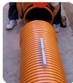
Left: SANECOR® pipe installation using discrete mechanical tools (medium and large diameters). Right: manual connection (small diameters)
