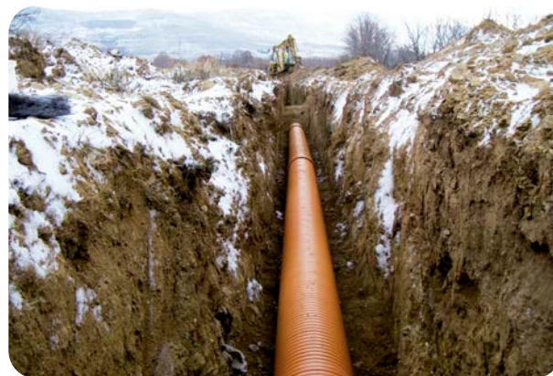
View of SANECOR® pipe installed in trench
