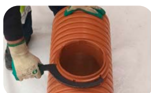
SANECOR® mechanical pipe clip installation
