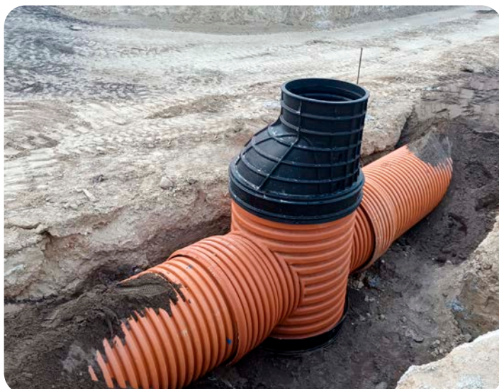
Installation of prefabricated welded manhole with solid base
