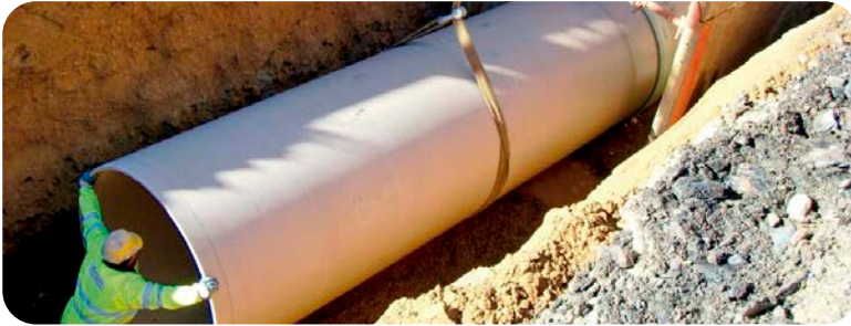
Installation of FRP pipes in a shored trench
