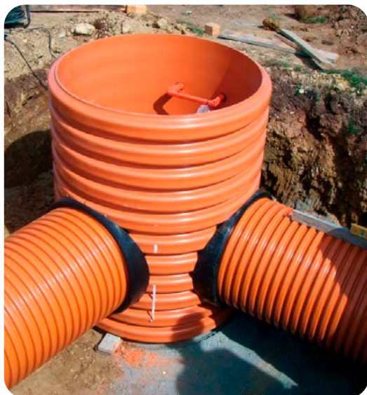
Manhole installation for pipes with direction change
