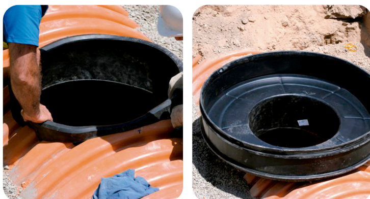
Installation of the body with inspection base
