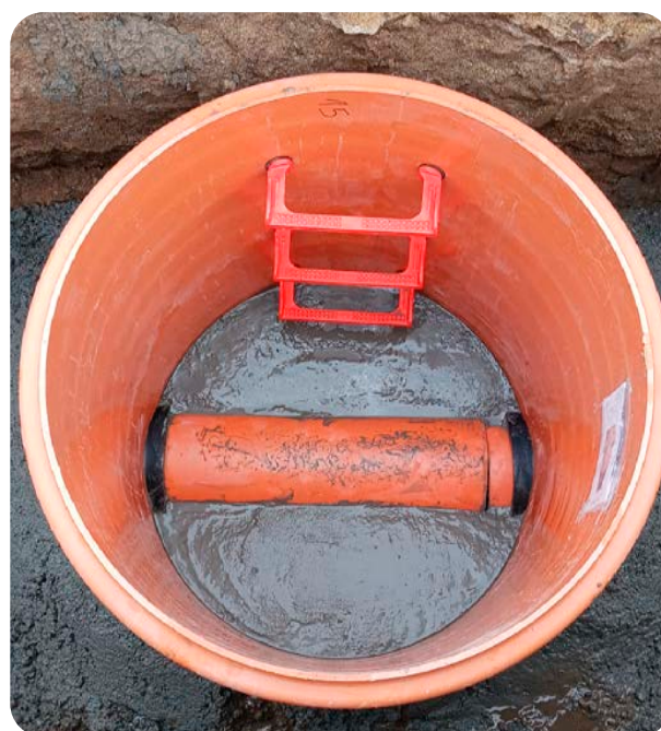
Concreting of the bottom of the SANECOR® manhole. 2nd phase
