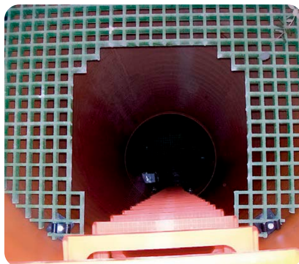
Polyester grating in SANECOR® manholes
