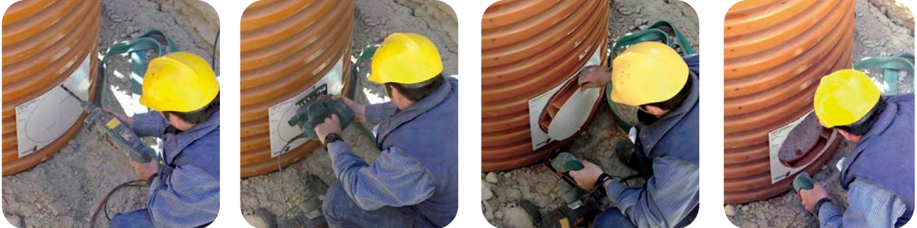
Drilling of holes for insertion of elastomeric clips
