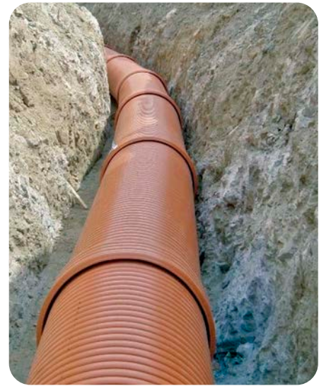
1,200 mm SANECOR® pipe with angular deflection
