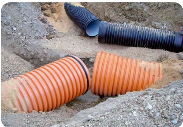
Corrugated PVC pipes (brick red colour) and corrugated PE pipes (black)
