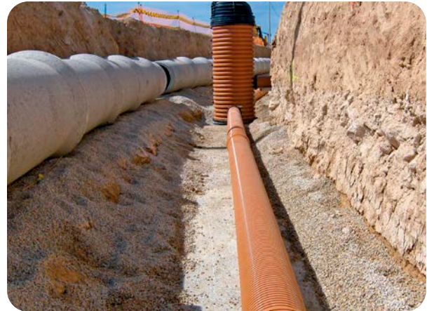
SANECOR® wastewater pipe and manhole and concrete stormwater pipe
