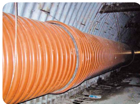
Installation of SANECOR® pipes in trench and in tunnel
