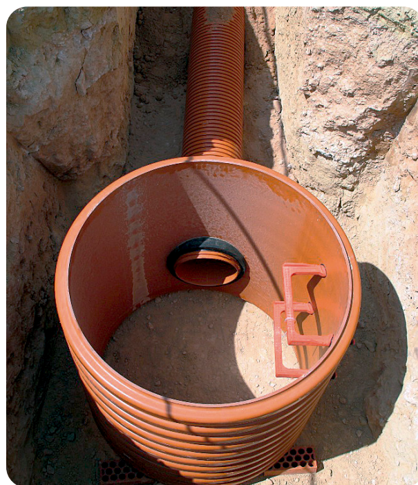
Concreting of the bottom of the SANECOR® manhole. 1st phase
