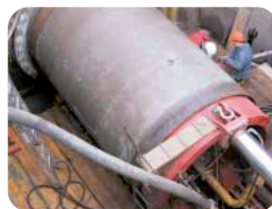
Polymer concrete (jacking pipes)
