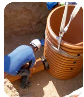
Fitting of pipes to the manhole body
