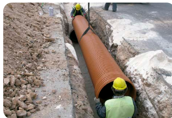
On-site handling of SANECOR® pipe
