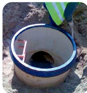
Manholes made of plastic materials (polyester and polyethylene)
