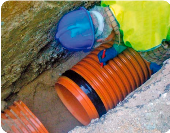
Manual connection of corrugated pipe
