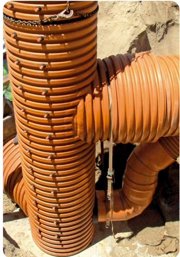
Drop manhole with SANECOR® manhole system
