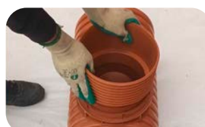
SANECOR® mechanical pipe clip installation
