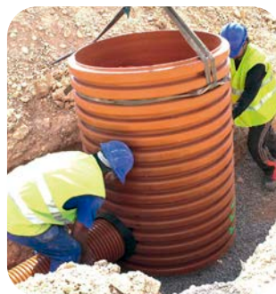
Fitting of pipes to the manhole body
