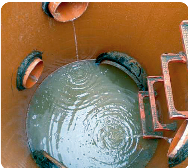
Multiple connections made in situ
