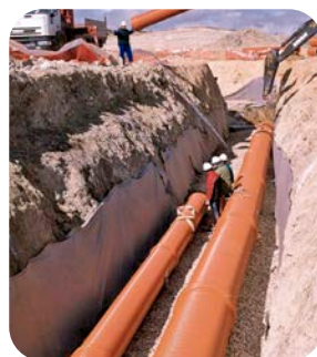
Left: SANECOR® pipe installation using discrete mechanical tools (medium and large diameters). Right: manual connection (small diameters)
