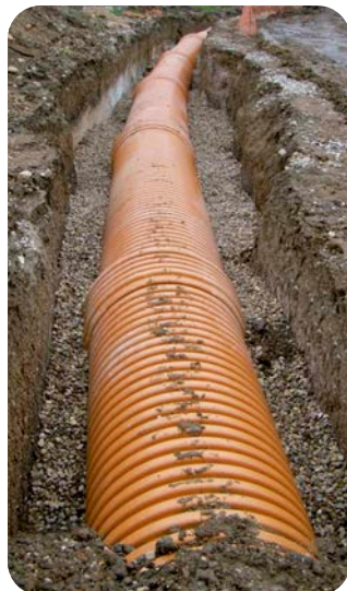
The flexibility of plastic pipes is important to absorb ground movements
