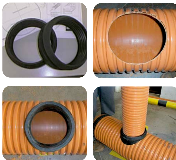
Elastomeric clips with cutting template for connections
