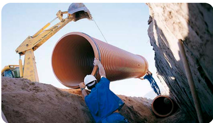
Installation of SANECOR® pipes in trench and in tunnel
