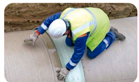
Sleeve joint on large-diameter FRP pipes
