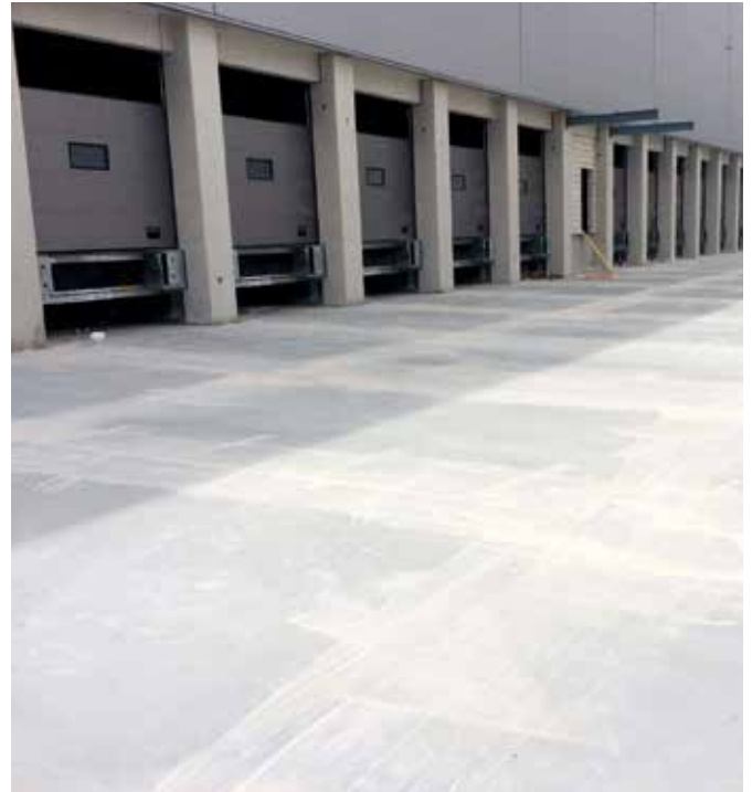
MasterFiber 246 Pavimento industrial, Madrid
