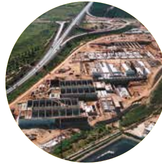
Desalination Treatment Plants
