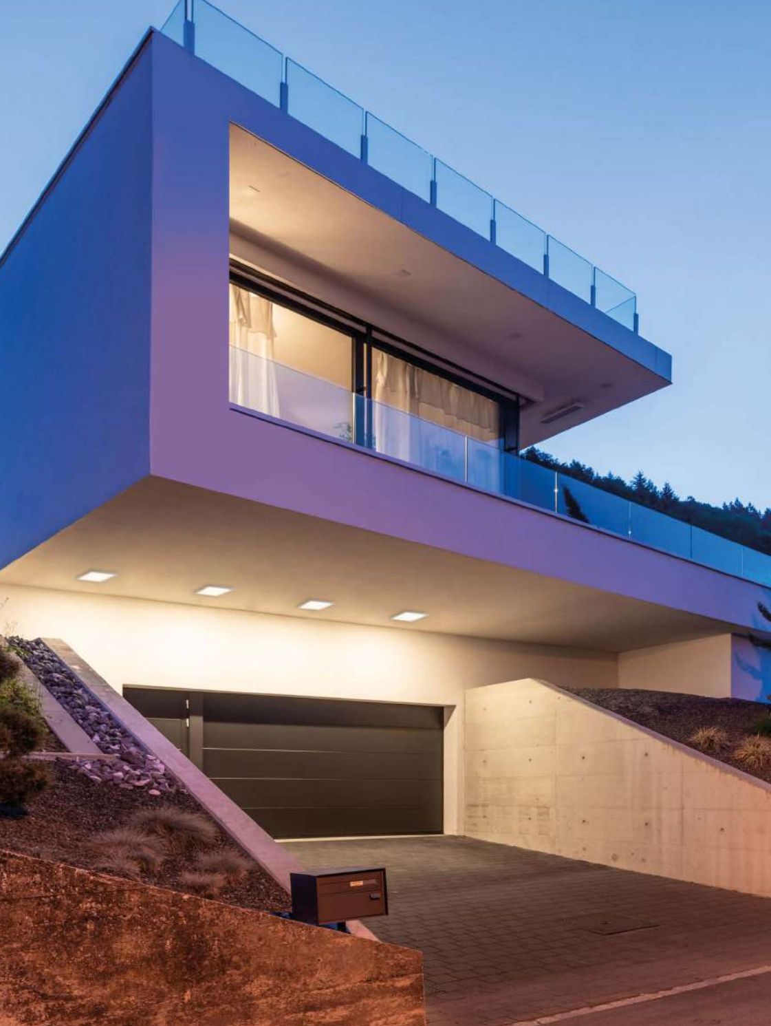
OUTDOOR - CEILING FIXTURES
