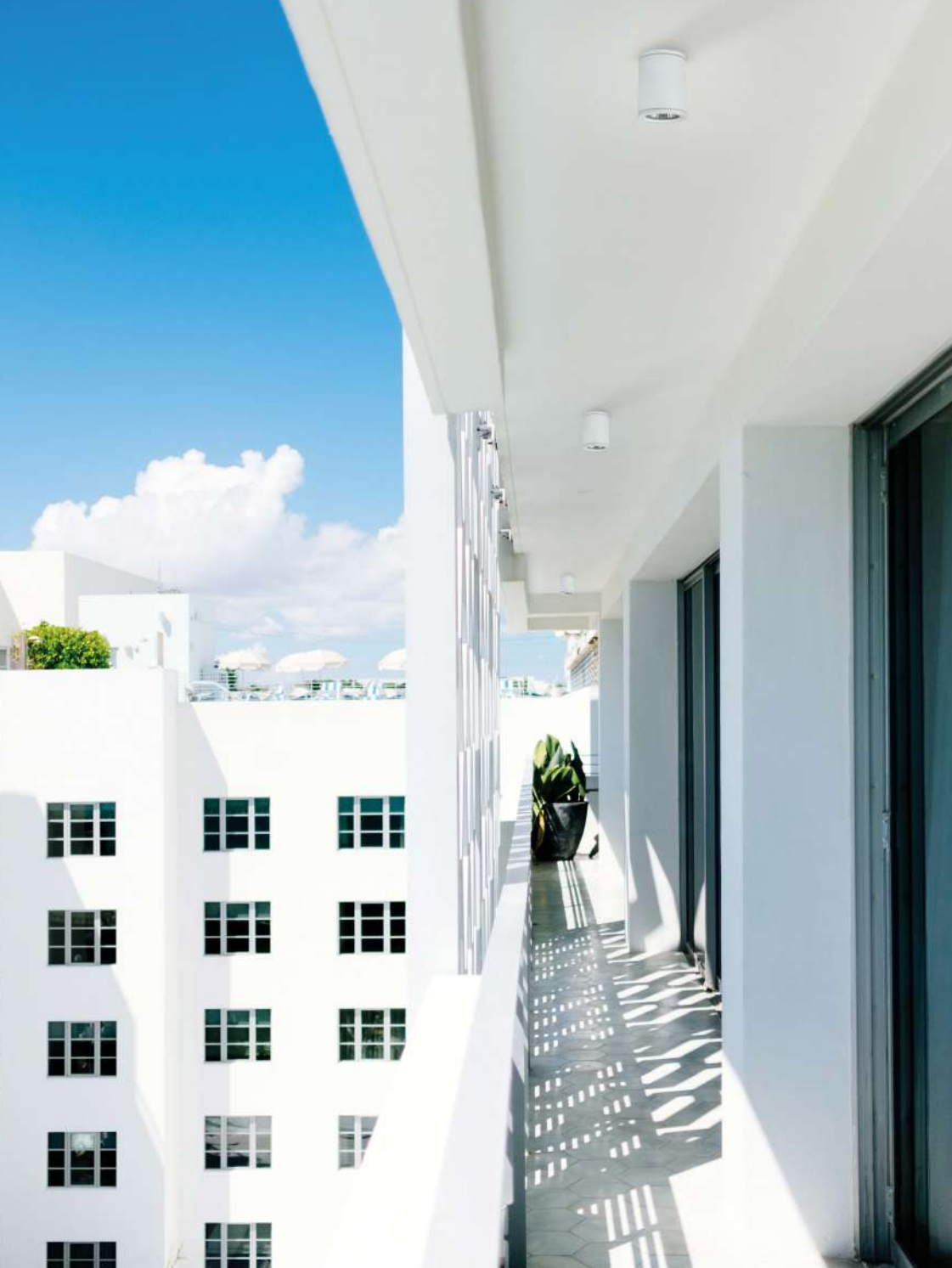
OUTDOOR - CEILING FIXTURES
