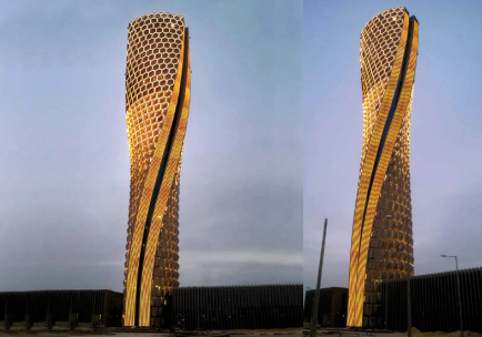
Doha Port control tower illuminated with LedFloodStrip®
