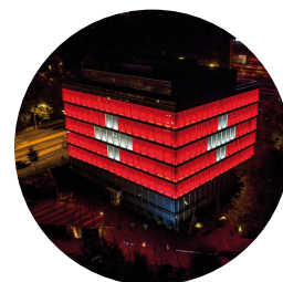
6 Amandolier Building SWITZERLAND
