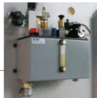
Centralina automatica per sicurezza idraulica Automatic station for hydraulic safety system
