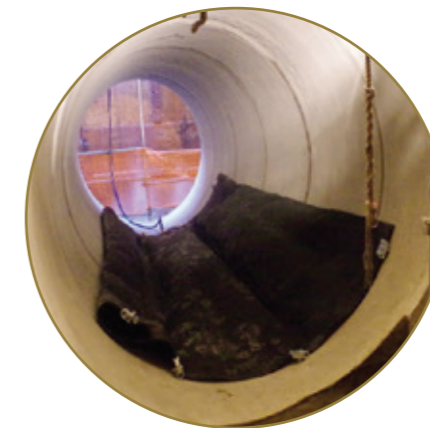
Placing – pillow plug should be positioned horizontally
