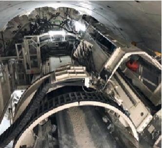
Brenner base tunnel Case Story
