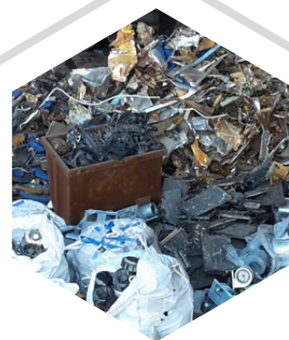
Waste from industrial demolition
